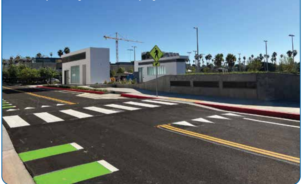
Two buildings that provide access to the underground Sustainable Water Infrastructure Project in Santa Monica are the only visible signs of the RO facility at ground level.
