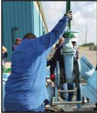
Spread outside flanges & remove old valve
