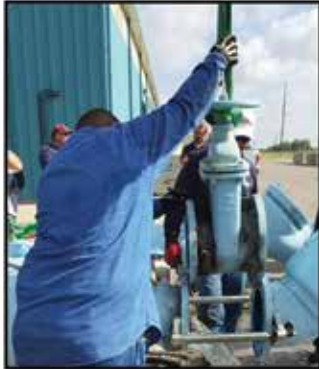
Spread outside flanges & remove old valve
