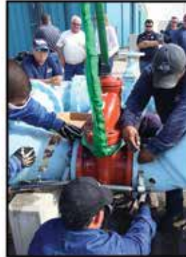
Reinstall new valve
